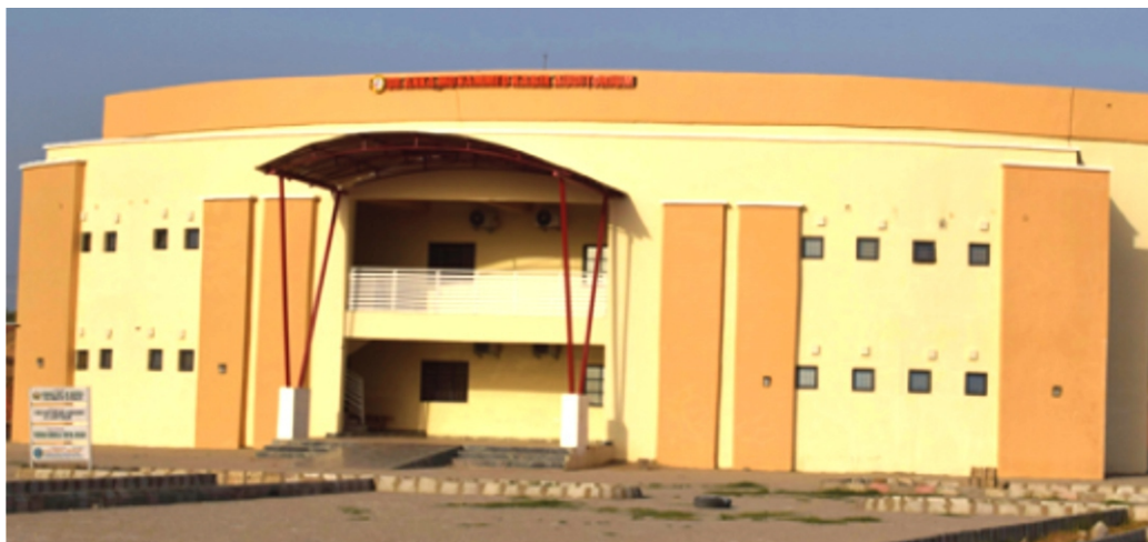
Front Facade view of Dr. Anka Mohammed Kabir Auditorium
